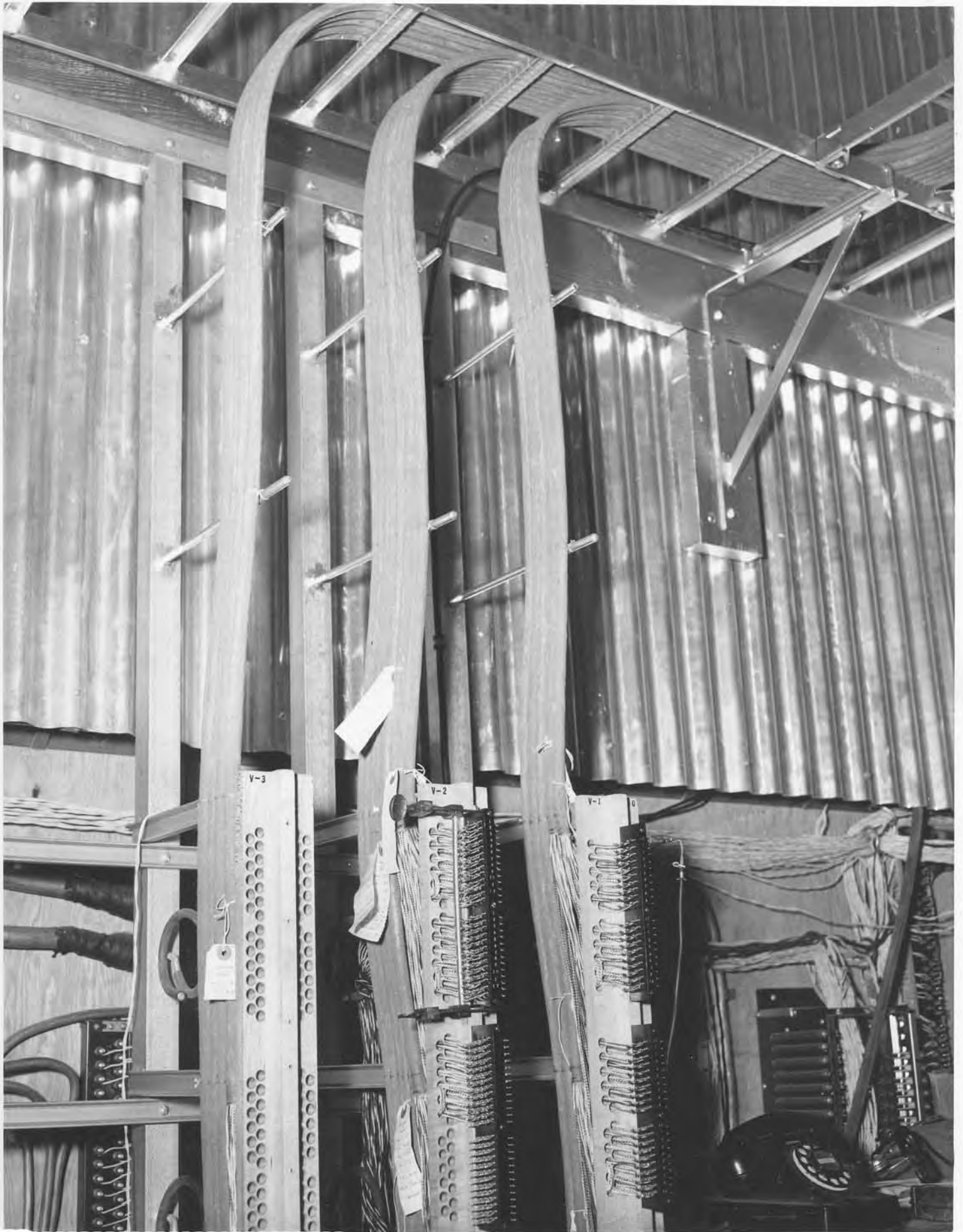
IDF, CABLE RUNS, KELLOGG 7-2 X-BAR, EDWARDS AIR FORCE BASE DOUGLAS AIRCRAFT, CA 1955
