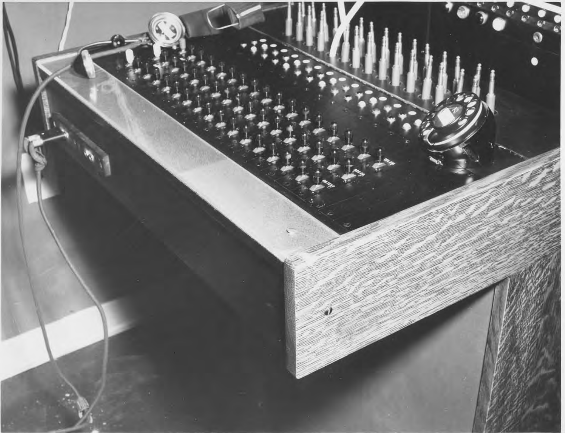
KELLOGG ATTENDANTS SWITCHBOARD, KELLOGG 7-2 X-BAR, EDWARDS AIRFORCE BASE, DOUGLAS AIRCRAFT, CA 1955
