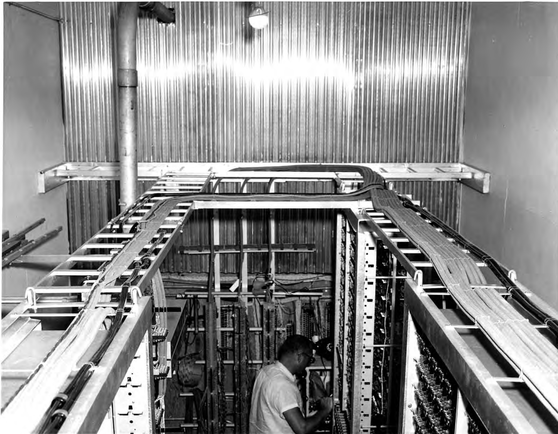
CABLE RACK WITH SEWED CABLES, ODIS LEVRIER TESTING KELLOGG 7-2, X-BAR, EDWARDS AIR FORCE BASE, DOUGLAS AIRCRAFT, CA 1955
