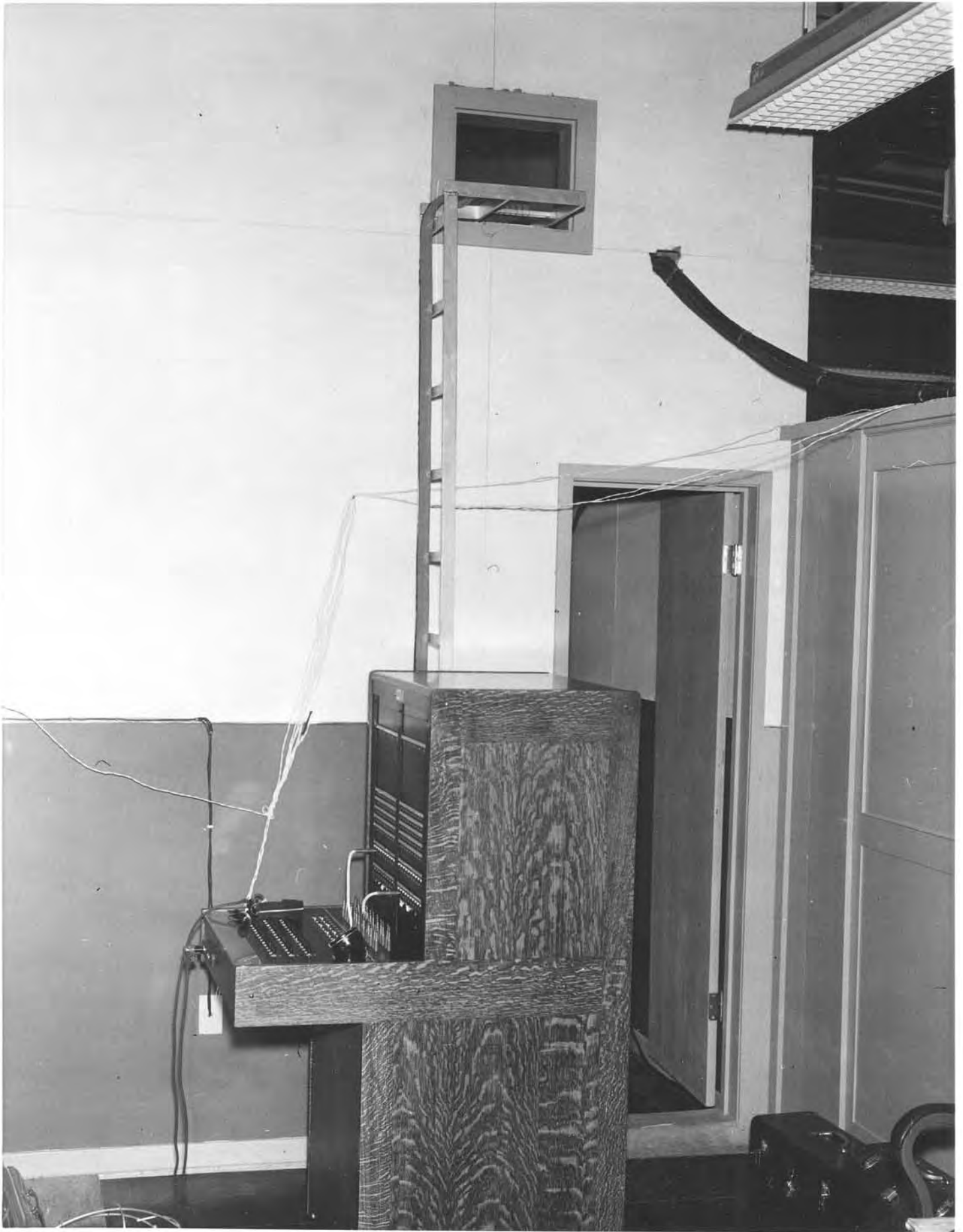
KELLOGG ATTENDANTS SWITCHBOARD, KELLOGG 7-2 X-BAR, EDWARDS AIR FORCE BASE, DOUGLAS AIRCRAFT, CA 1955
