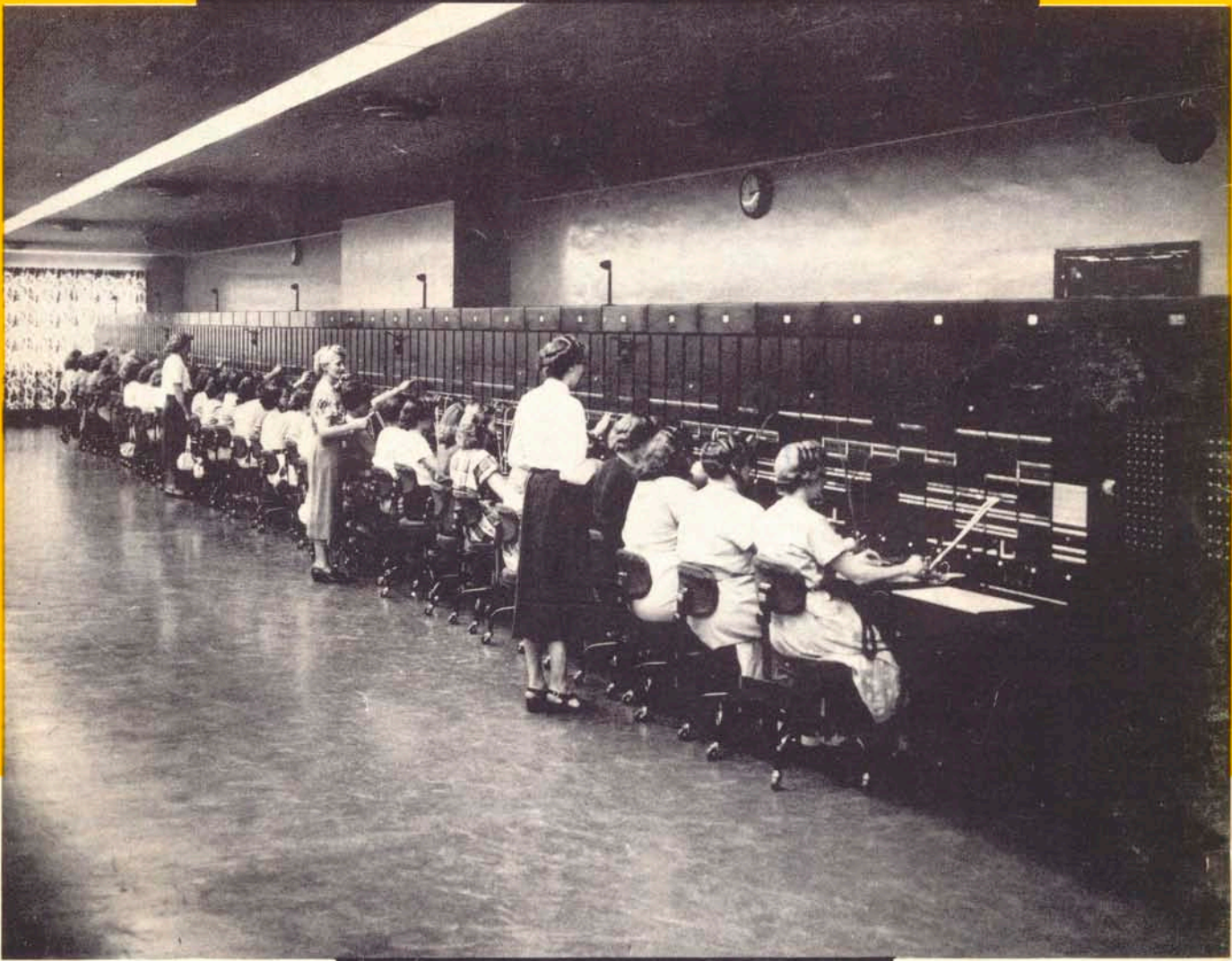
WARREN, OHIO KELLOGG 3C TOLL SWITCHBOARD
