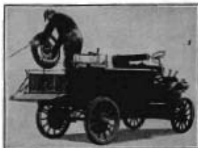
No. 4609-104 Reel Applied to an Auto Truck
